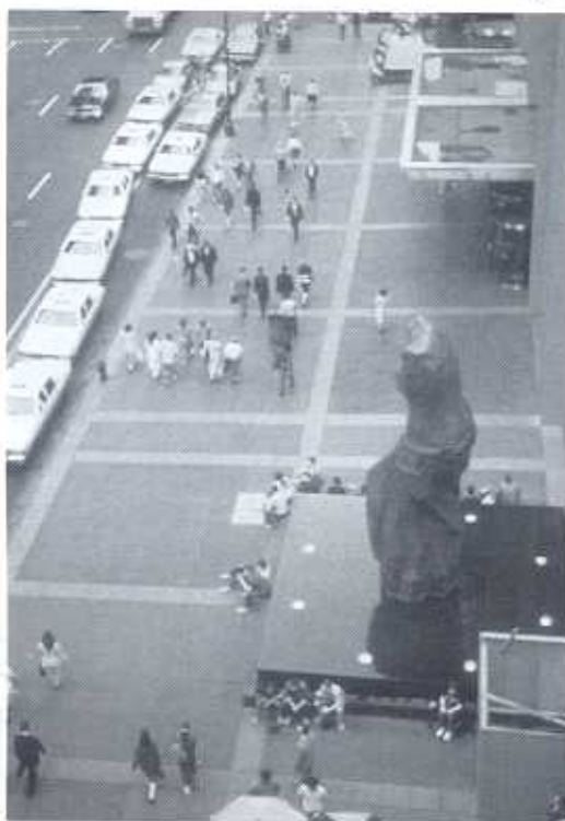
At the Credit Lyonnais Building, 1301 Avenue of the Americas in New York, single unit pavers allow for grid patterning. (photo: L.M. Scofield Co.)
