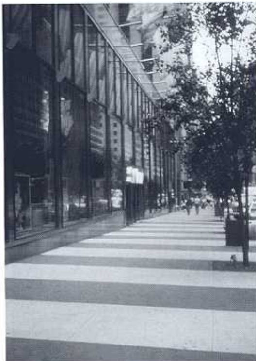
Uncolored concrete, and a dark gray colored concrete in a sponge float finish, were used at the Daily News Building in New York. (photo: L.M. Scofield Co.)
