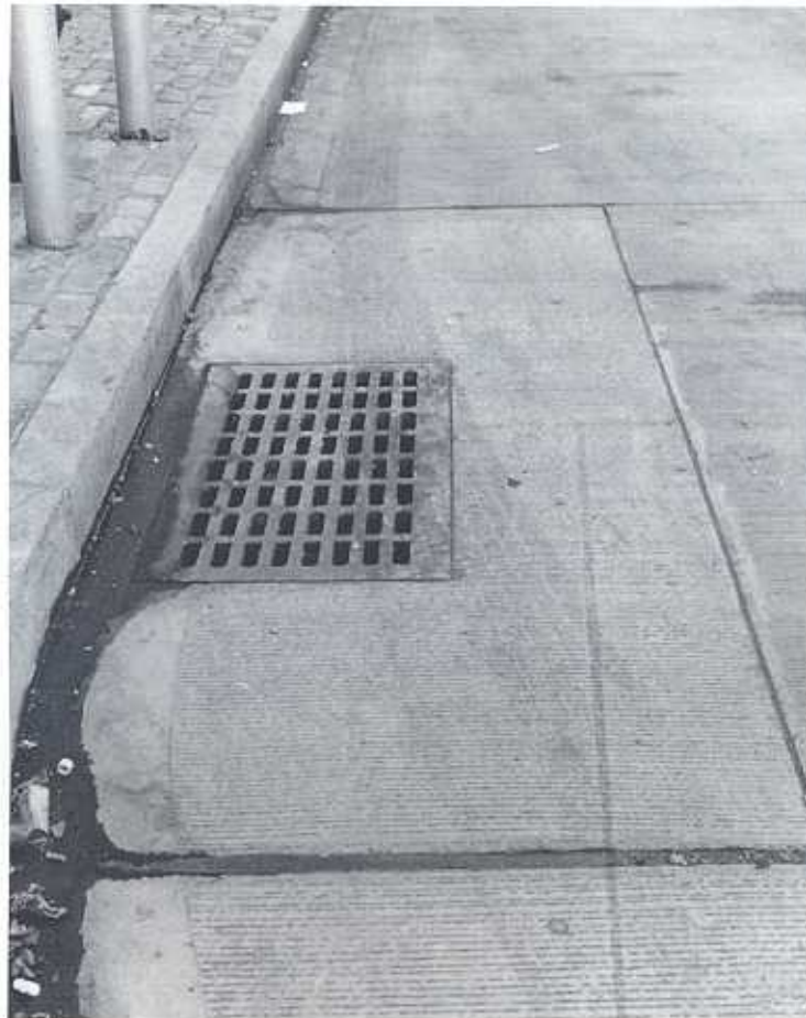
Figure 5 and photo below: Catch Basin Isolation
