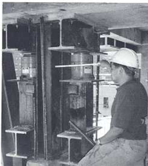
Photo 3: Checking placement of hydraulic jack.
