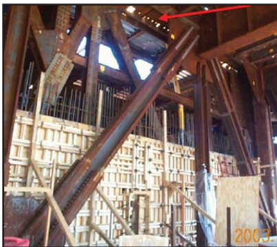
Figure 8. 731 Lexington Avenue - Transfer truss about to be encased.
