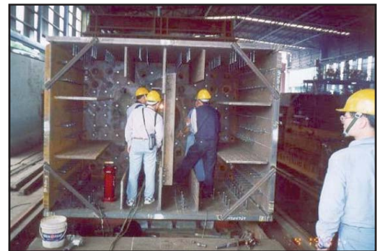
Figure 10. Taipei 101 - Super-column fabrication.
