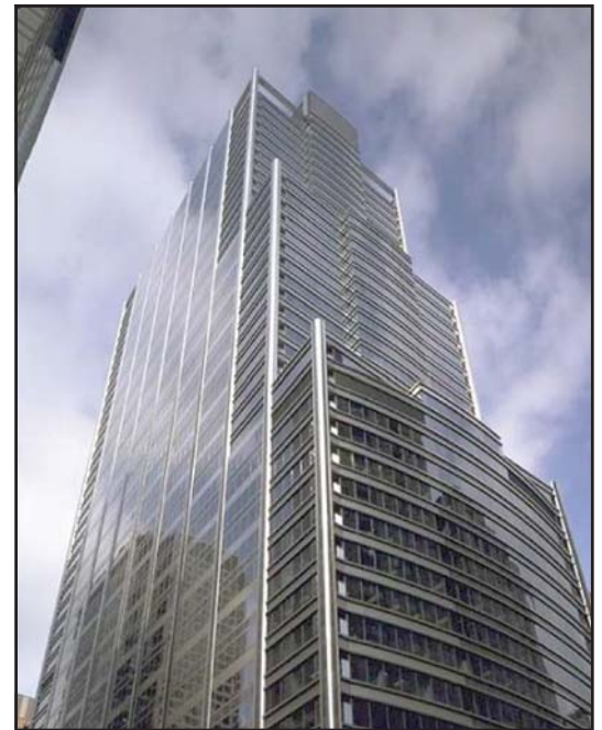
Figure 2. UBS Tower - 50 stories, concrete core, steel frame.
