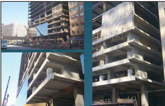
Figure 6. 191 North Wacker - Stepped sloping concrete columns.
